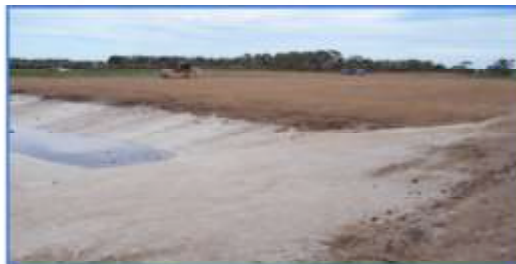
Abattoir waste composting site & holding dam
